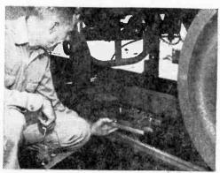
The support crank arms for the sensor assemblies ride at speeds up to 157 mph, ¾ of an inch above the track on a test train. By measuring the capacitance across the air gap between sensor and rail, the sensor assemblies act as proximity detectors, measuring horizontal and vertical rail alignment, track gauge and superelevation.
